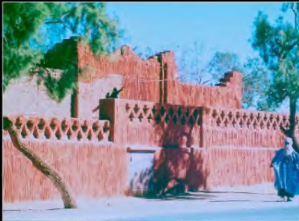
All buildings were of mud. This one is having a new layer applied
