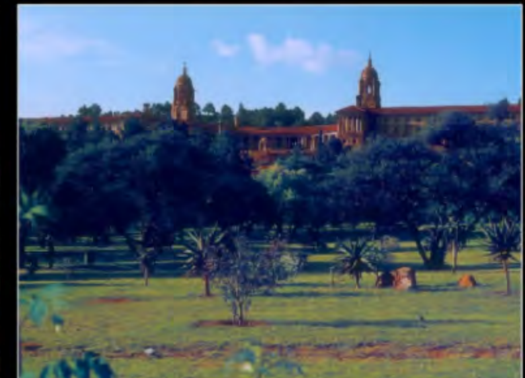
Parliament buildings - Pretoria is administrative capital but Capetown has the legislature. All the government moves to Capetown for 6 months of the year
