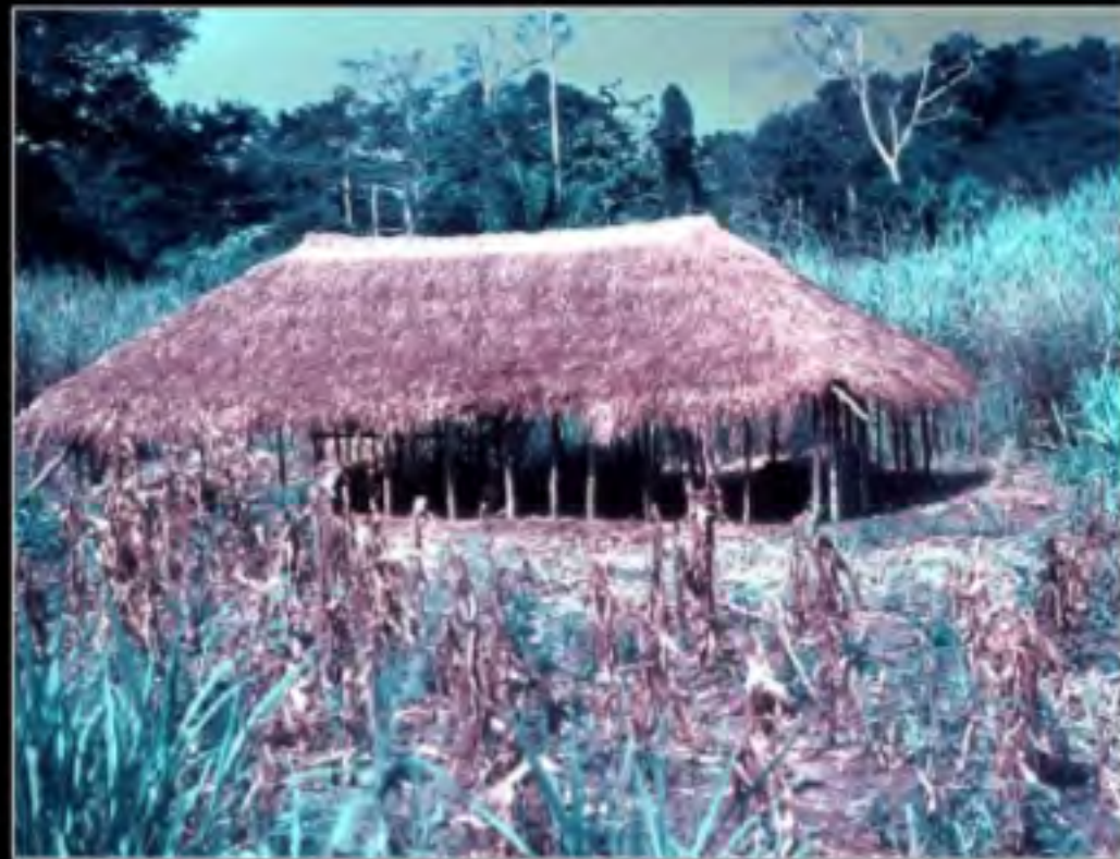
A deserted house - built of local materials
